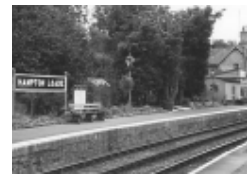
The south end of Platform 1
